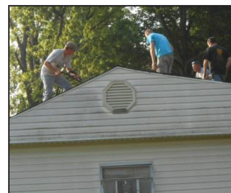
Pictured from left to right are Anthony Losekamp (Berco Construction), Casey Knigga (Casey's Outdoor Solutions), TJ Jacobs (Berco Construction) and Jason Cox (JDC Construction).
